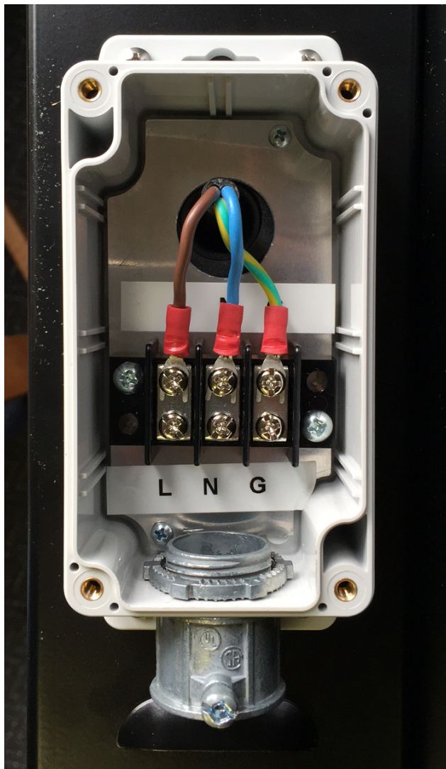
Figure 6 - Cover removed from NEMA watertight junction box.
