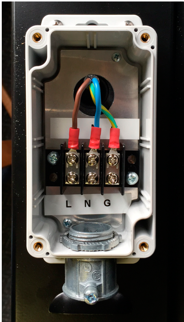
Figure 2 - Cover removed from NEMA watertight junction box
