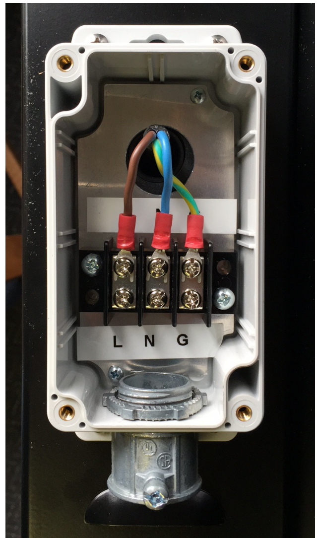
Figure 7 - Cover removed from NEMA watertight junction box.
